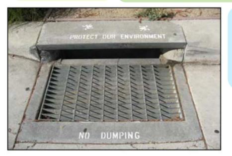
Runoff can also collect contaminants from roads carry them into our drainages. Proper storm water runoff management eliminates the possibility of impacts on storm water quality. Do NOT discard anything on the ground!
